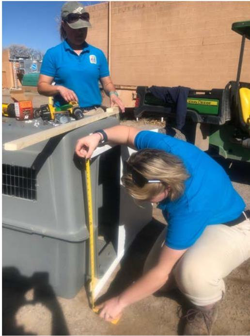
7. Cut your door material (FRP or PVC sheeting) to the correct size. Determine which direction you will want the door to slide and attach scrap wood or plastic to the door to create a handle. The handle will also stop the door from sliding completely off in one direction.
