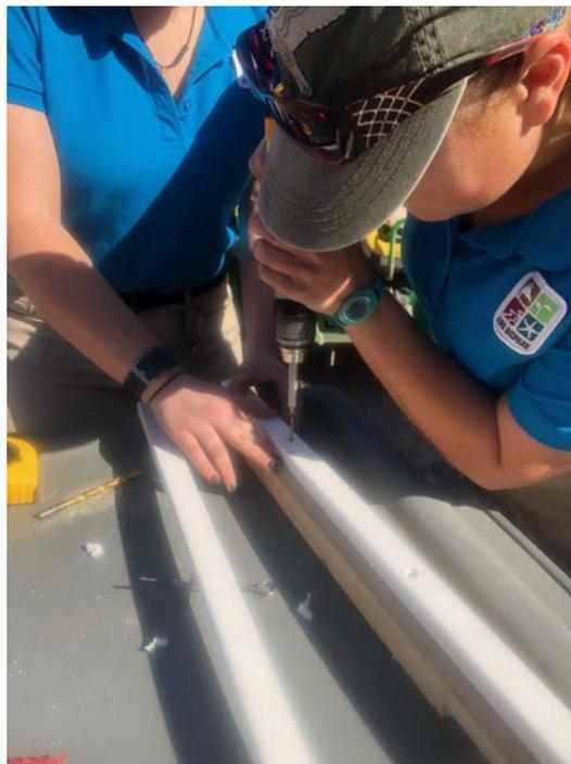
4. Attach the track to the crate now, placing the wood/lattice cap track in the center on the top of the crate. Depending on your type of wood and screws, you may want to drill pilot holes into the wood in the locations where the wood will line up with the crate holes.
